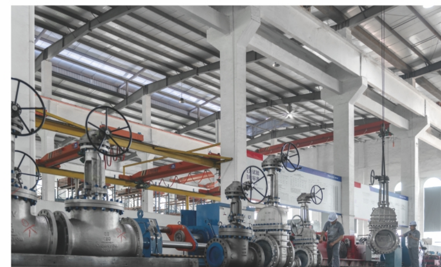
• 试压检测 Pressure Test & Inspection
